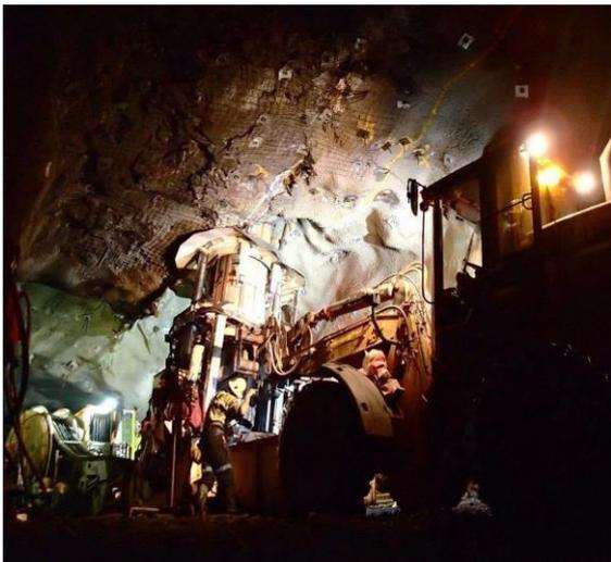
Figure 4. Installation of the BBM with pipe change
