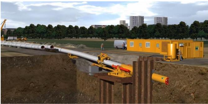
Figure 9. Direct Pipe method with slurry MTBM and Pipe Thruster in launch pit.
