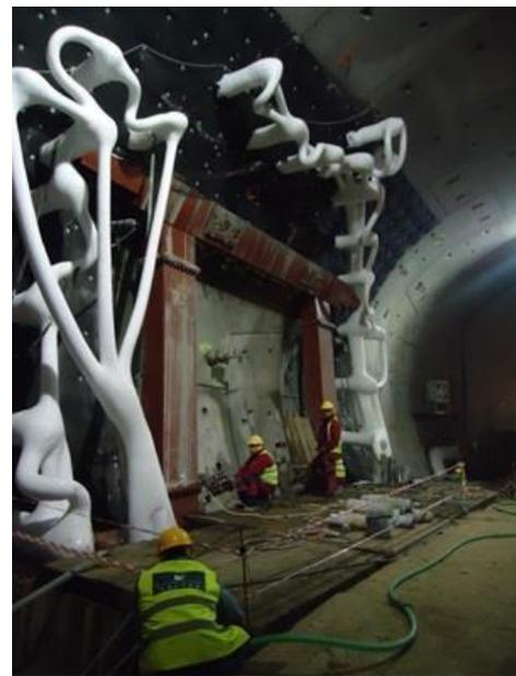
Figure 26. Cross-passage excavation in road Gdansk (Poland) Tunnel under Vistula River. Freezing pipes and steel frame to support ring opening.
