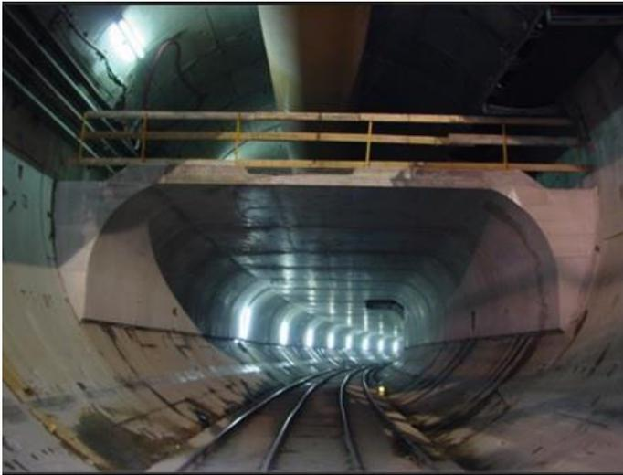
Figure 33. Cast-in-situ middle slab for L9 metro line in Barcelona.
