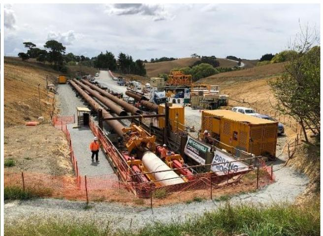
Figure 14. 48" Direct Pipe® going for 2,000m record drive at Snells Algies.
