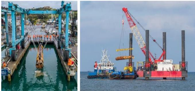
Figure 11. Direct Pipe recovery options – land based lifting versus jack up platform, UK.
