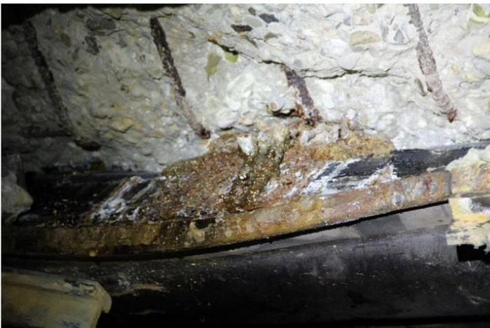
Figure 15 - Gina seal pushed inwards due to soil buildup
