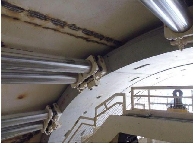
Figure 8 Thrust pads to segmental lining (Riyadh Metro TBM).
