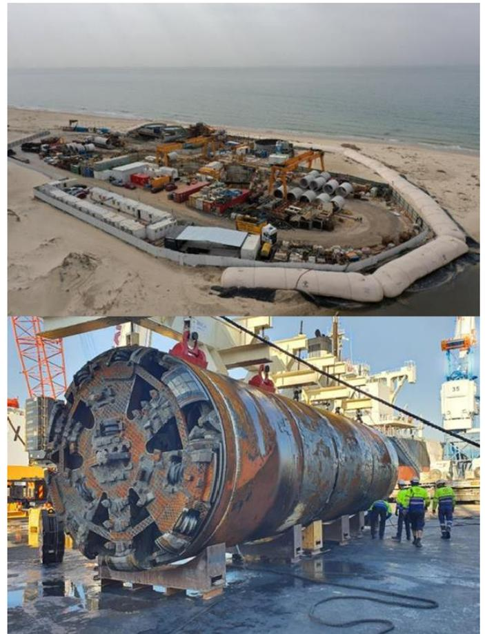
Figure 4. Sorek II pipe jacking jobsite and upskinned AVND2000 after recovery in harbour (Eurohinca).
