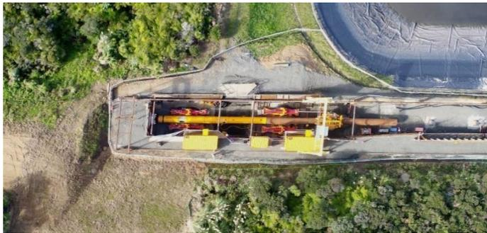
Figure 13. AVN1000DP for 48" pipeline and 2x Pipe Thruster installed in the launch pit onshore.
