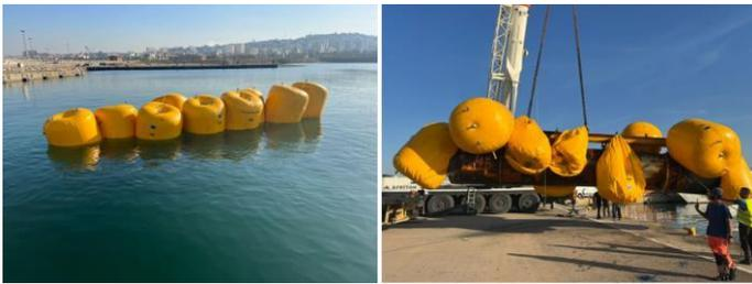
Figure 3. Lifting of AVN1200 with airbags, El Marsa desalination project, Algeria (RADCO SARL).
