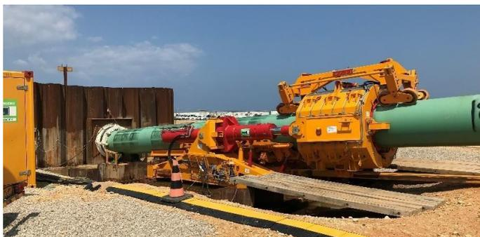
Figure 12. HK750PT Pipe Thruster pushing forward the 56” gas pipeline.
